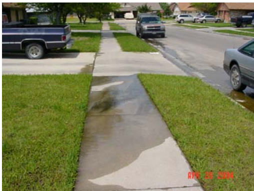
Groundwater seep flowing over sidewalk
